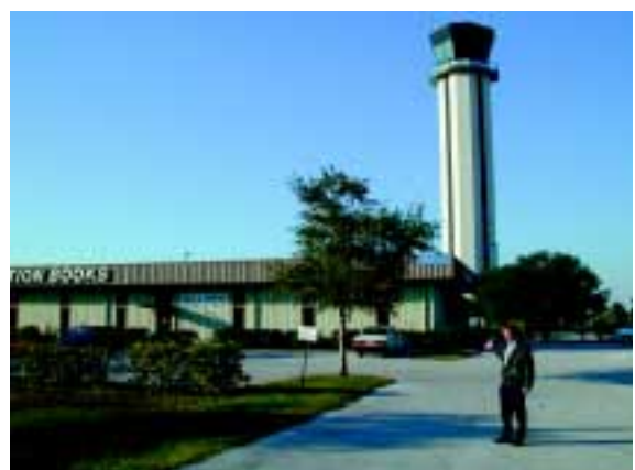
Office building at the apron of the airport, in front S. Unzicker
